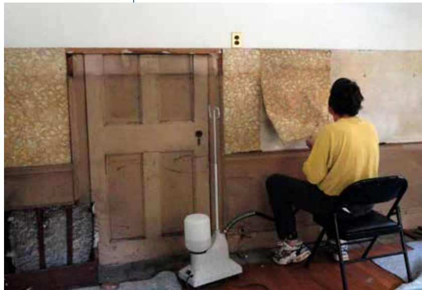
Figure 3. History Revealed. Wallpaper installed in 1883 was uncovered behind a late-19th century bookcase in the family's library at Fairsted. Here the fragments are being removed for conservation and reproduction by a Studio TKM conservator. Note the corresponding woodwork's historic decorative paint treatment. Photographed by Carole Perrault, November 2010.
