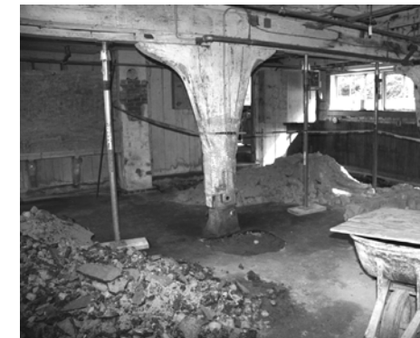
The barn at Fairsted will become a focal point for Good Neighbors activity. Photo by Jean Stringham
